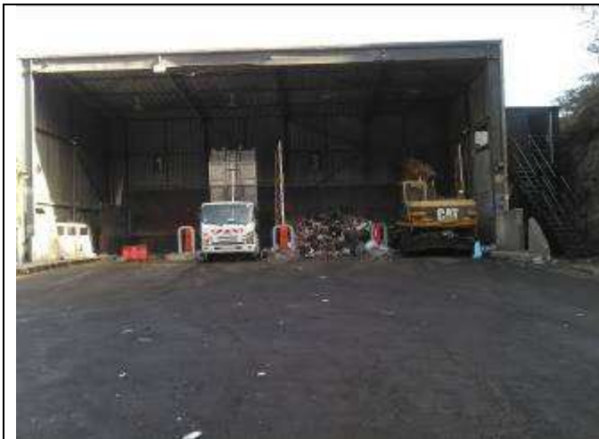
Quai de transfert (4 trémies)
